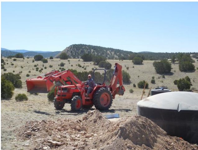
Working on Solar Well Storage Tank
